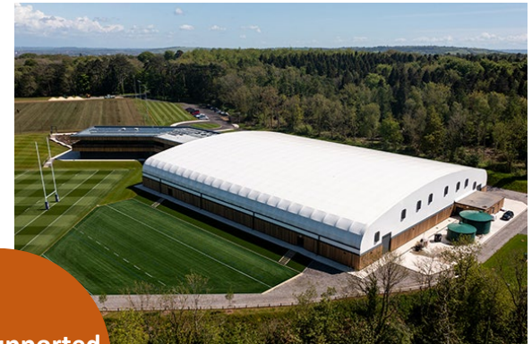
Frame Supported Fabric Building
